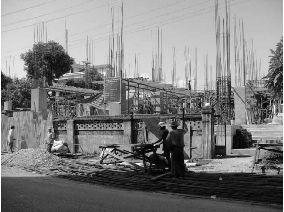
Construction site in Yangon
